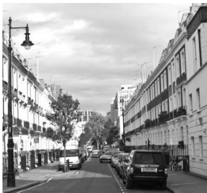
Figure 6: General view of Hugh Street, Pimlico
